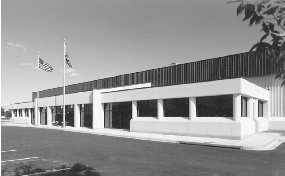
FIGURE 7.35 Precast wall panels add depth to the façade. (Photo: Maguire Group Inc.)
